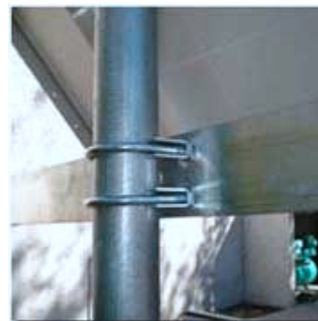
Side of pole solar mounting structure U bolt attachment
