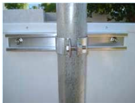
attachment with Unistrut clamp
