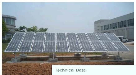
Installation Site: field Open Wind Load: Up 60m/s Snow Load: 1.4KN/m Applicable Module: Framed or Frameless Module Orientation: Portrait Main Material: 100% Anodized Aluminum Fastener Material: Stainless Steel
