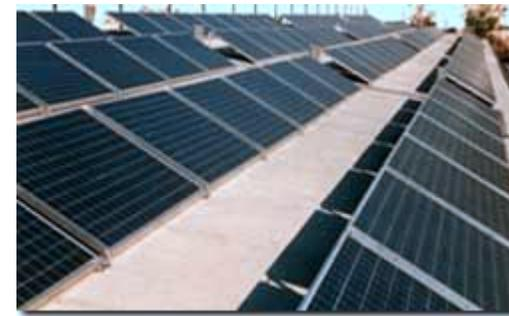
Wedge Mounted Solar Power Array
